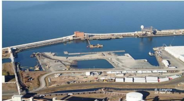
Port of Belledune Ro Ro Barge Terminal
