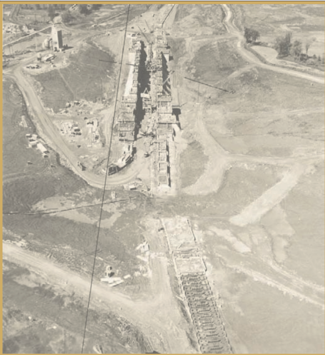
Long Sault Canal construction, May 16, 1957.
